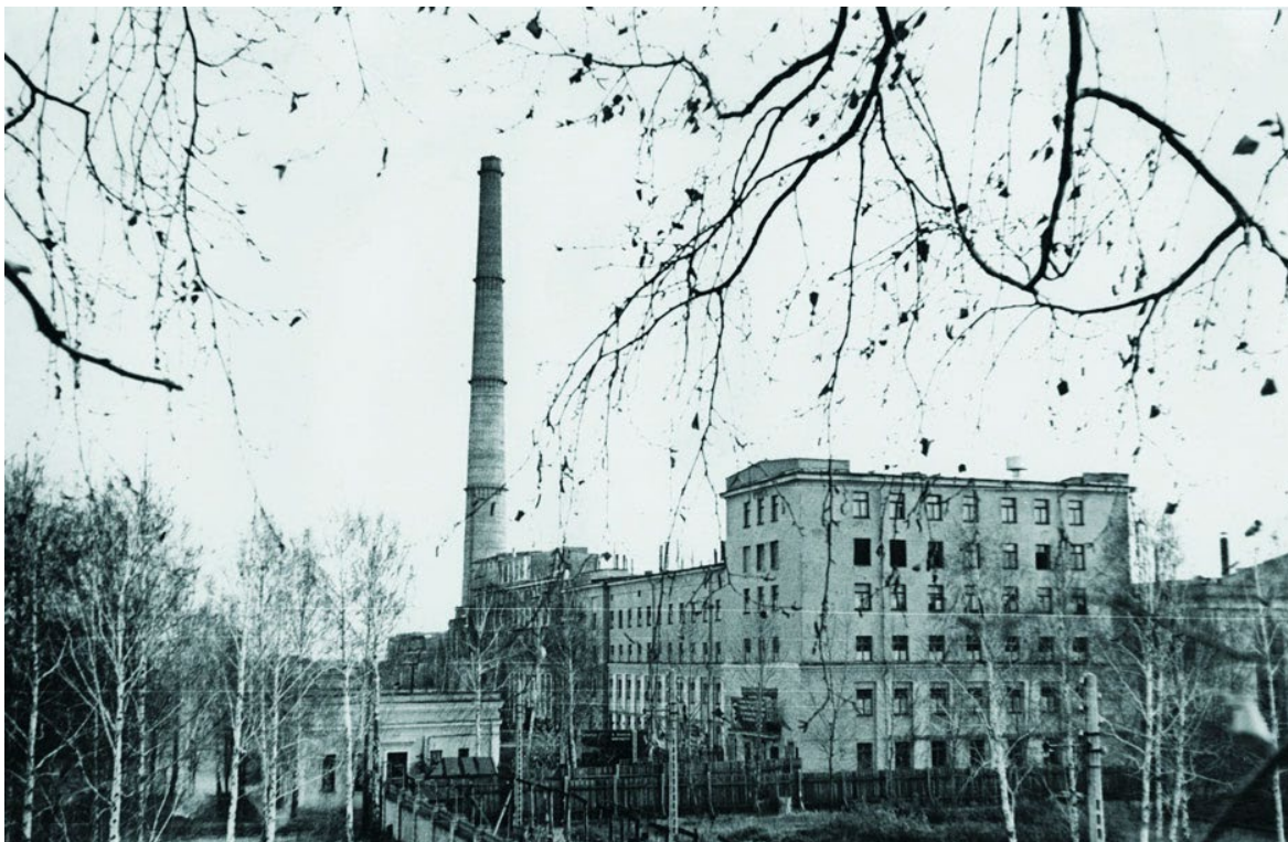
Figure 15. First plutonium separation facility at Mayak in 1948
